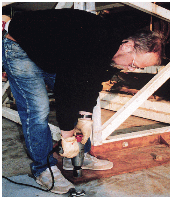
Figure 7: Securing Winch to Deck
