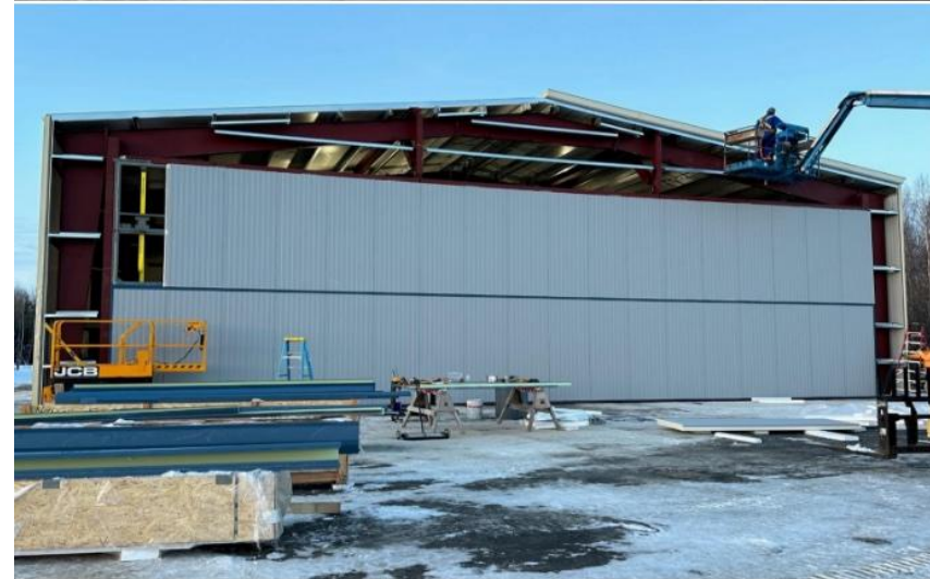
AWIP Panels on garage door
