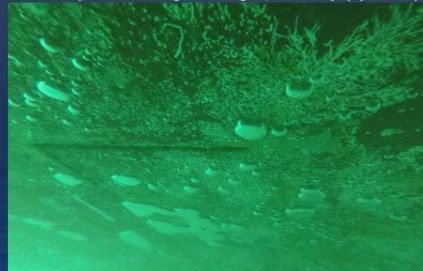
Diver inspection showing biofouling on/near arrays (April 2023)
