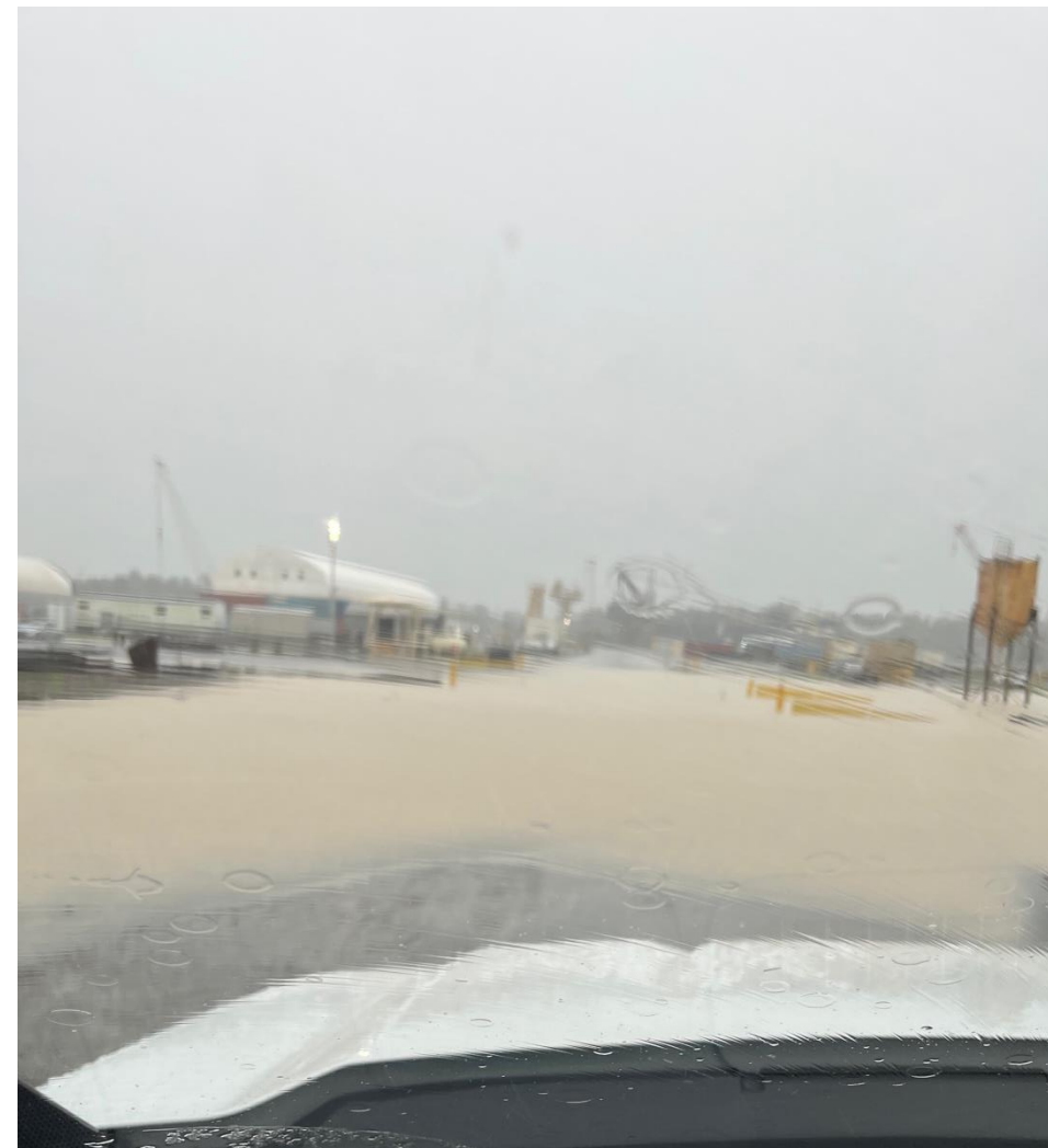
Houma Shipyard Flooding
